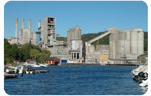
The Norcem cement factory at Brevik in Norway (Photo:Norcem)
